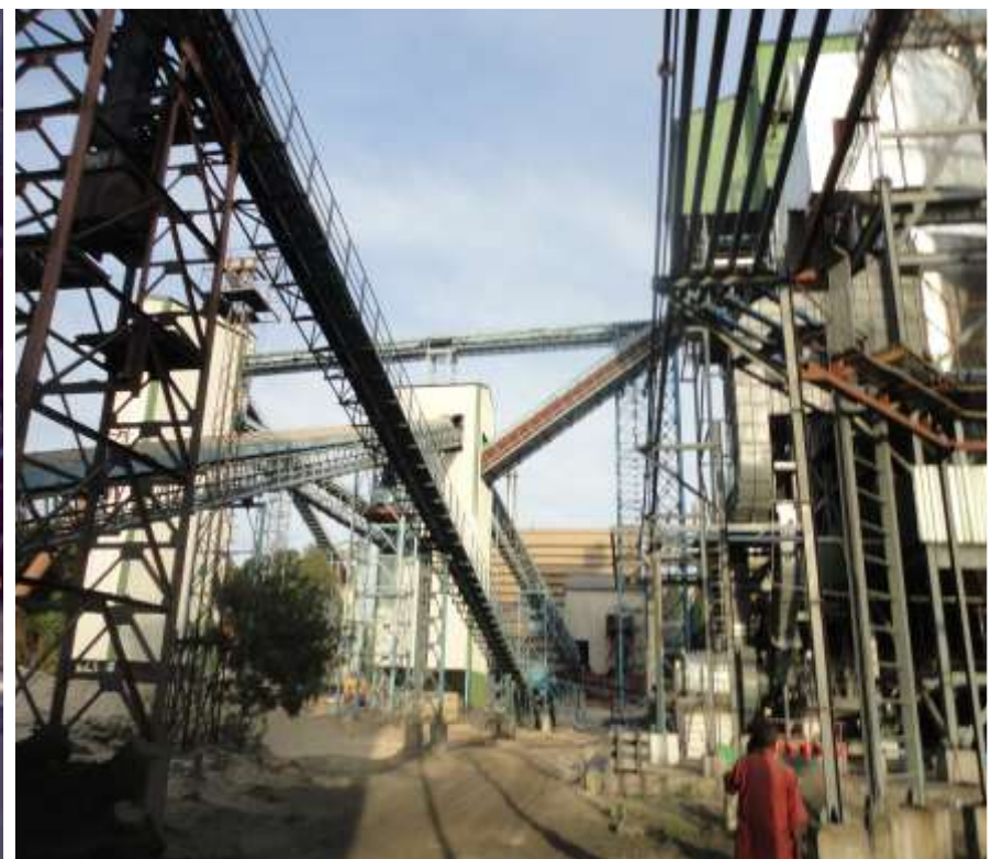
Bagasse, Coal & Ash Handling System At Ponne Sugars
